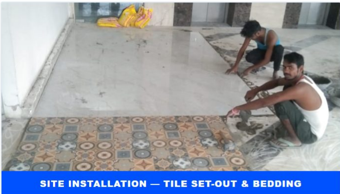
SITE INSTALLATION — TILE SET-OUT & BEDDING Active layout, joint spacing and manual bedding of large-format tiles and decorative floor inlays.
