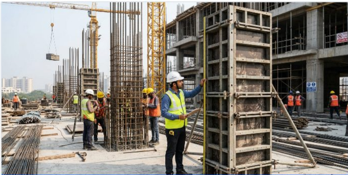
CIVIL WORKS • REINFORCED CONCRETE
