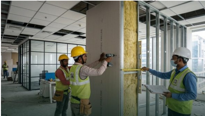
PLATE 02 // ACOUSTIC PARTITIONS & WORKPLACE FIT-OUT
